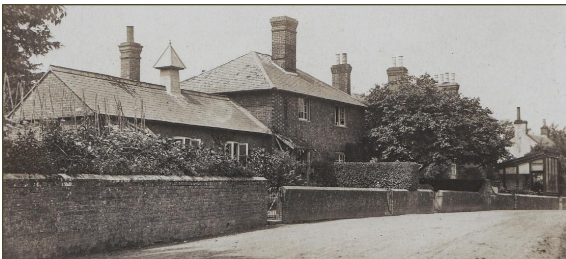
The school building in about 1918, later demolished for the building of the Oldaker Road housing development
