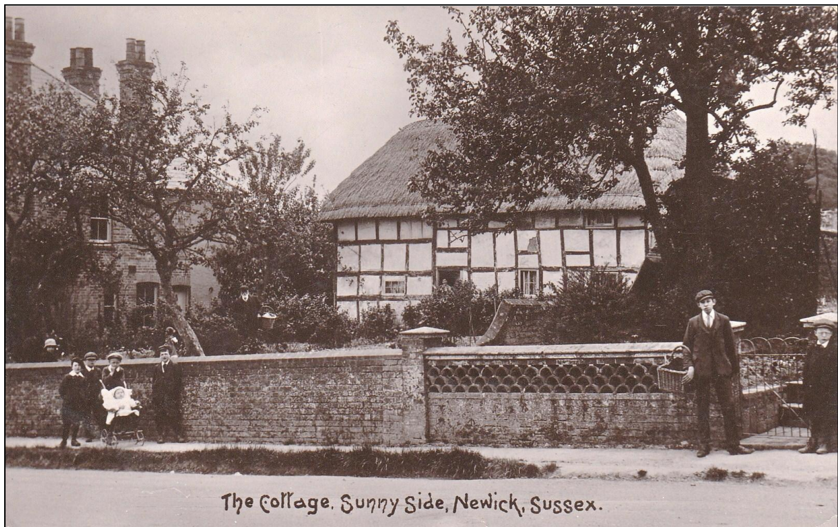
'The Cottage' in the High Street, Newick
